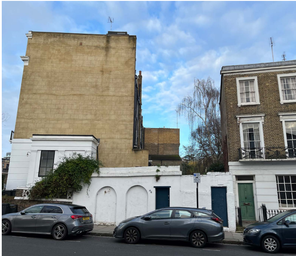
Existing View from Inverness Street
