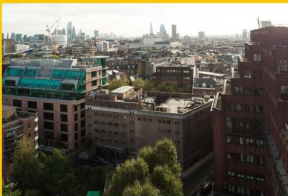
135 Shaftesbury Avenue Rear View
