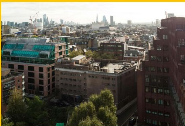
135 Shaftesbury Avenue Rear View
