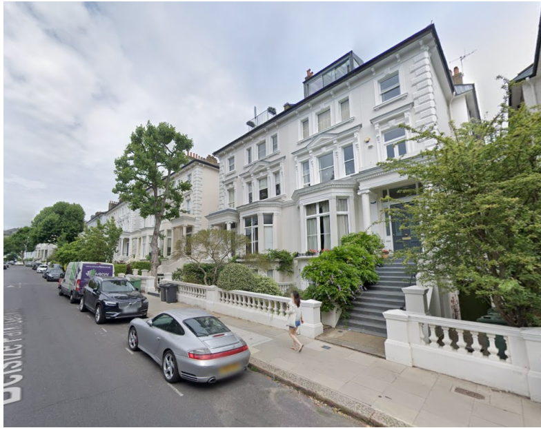
Above; Existing Street Elevation - Viewed from Belsize Park Gardens looking North West.
