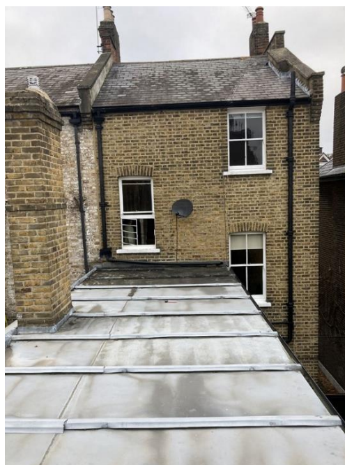
Image 1 – Existing chimney protruding from the two storey outrigger
