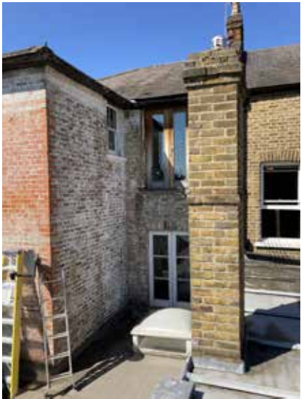
No.38 from Rear Outrigger roof
