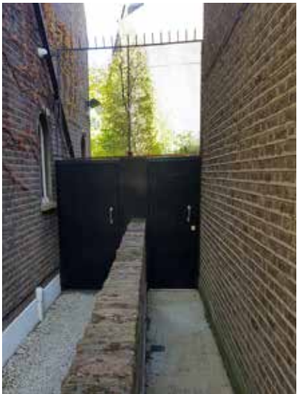
Existing side passage with No 34
