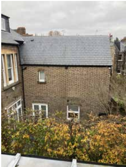
No.34 from Rear Outrigger roof
