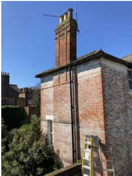
No.38 from Rear Outrigger roof
