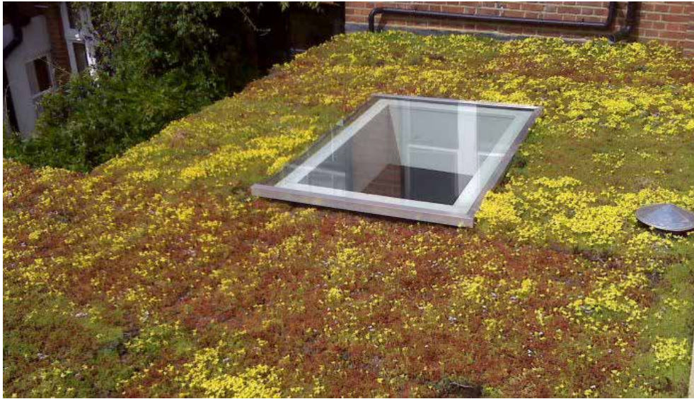
Extensive sedum roof covering
