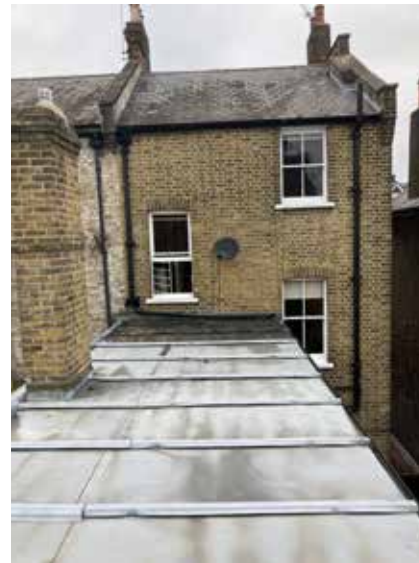
Rear elevation from rear outrigger roof
