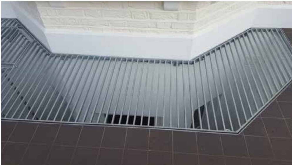
Grille to lightwell by bay
