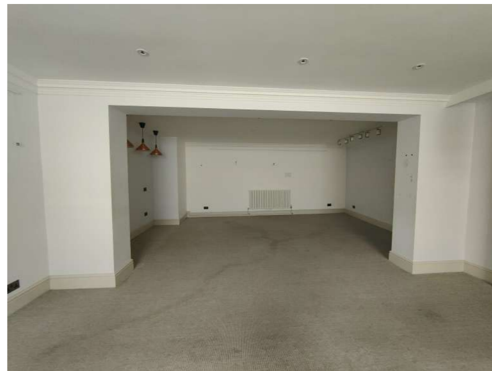
Figure 14: Conjoined basement room in house
