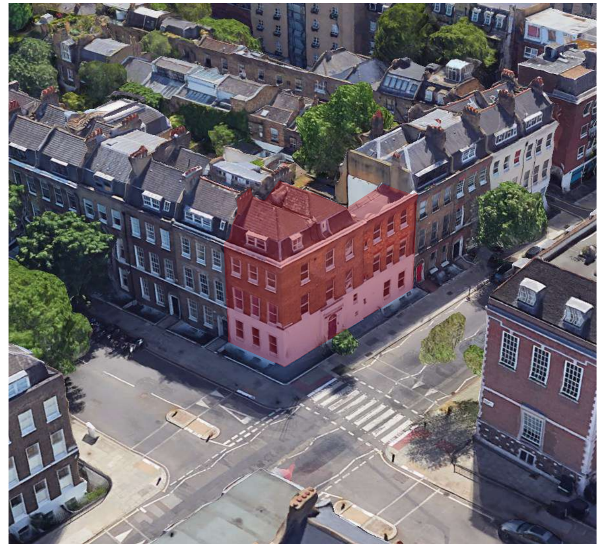
Figure 1: Aerial view of 8 Guilford Street, shaded red, and environs.
