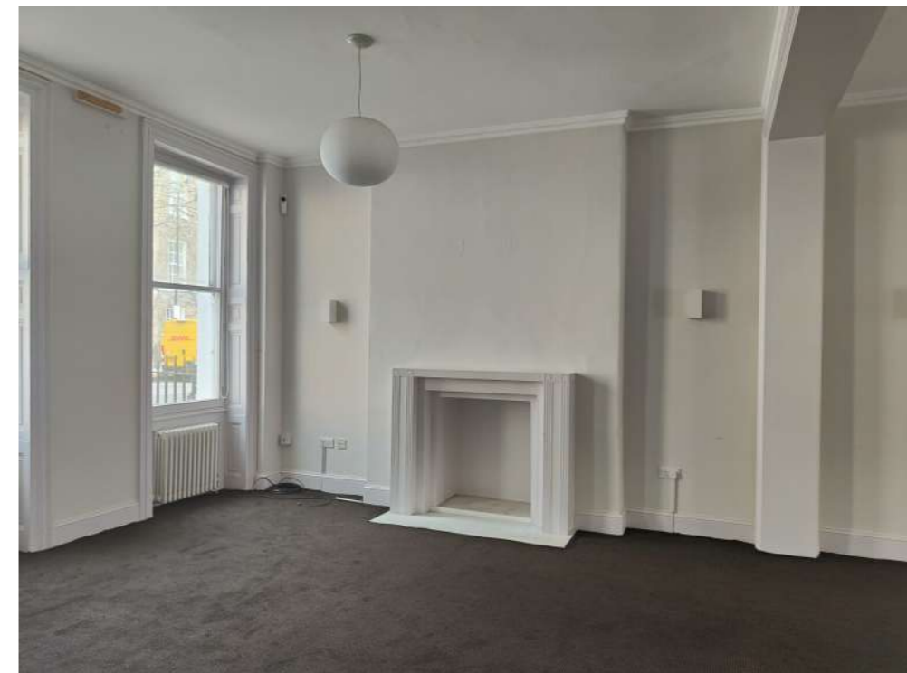
Figure 6: The same room today, note loss of historic fire surround, coving, dado rail, picture rail and skirting.
