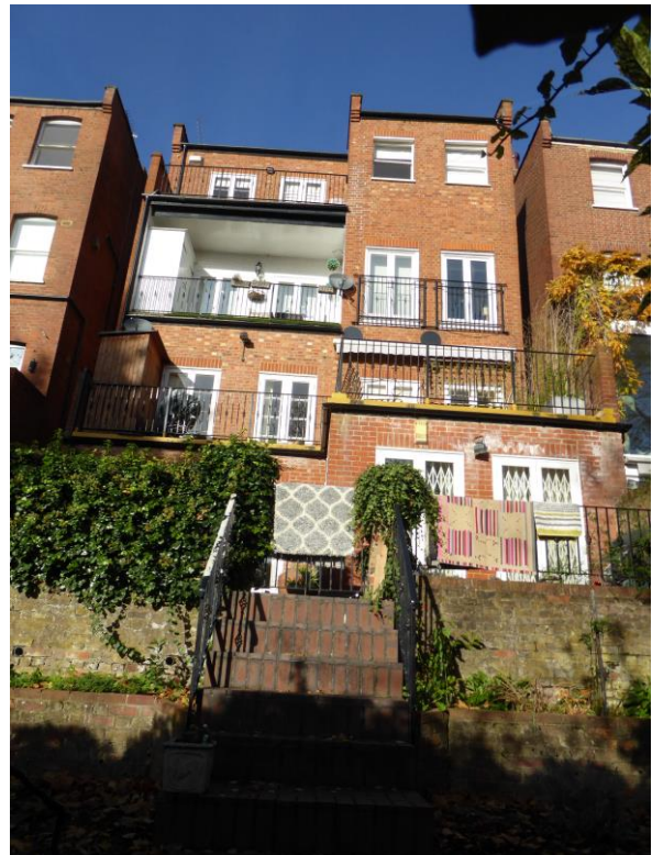
View of the rear elevation of at 4 Frognal Lane. The proposed external terraces proposed are heavily influenced by this existing arrangement.
