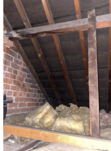
Existing loft insulation
