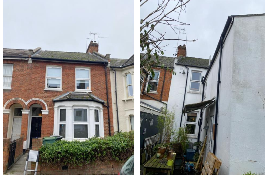
Existing windows and doors
