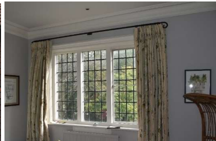
Single glazing 1 st Floor bedrooms exterior and interior views.
