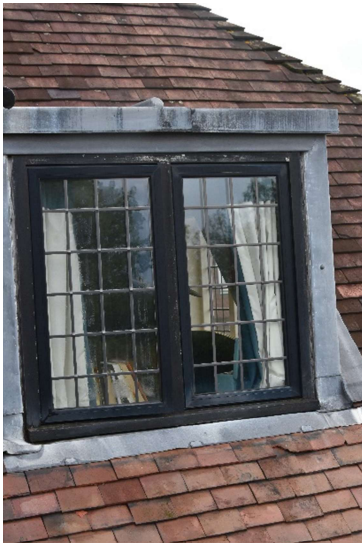
2 nd floor double glazed units
