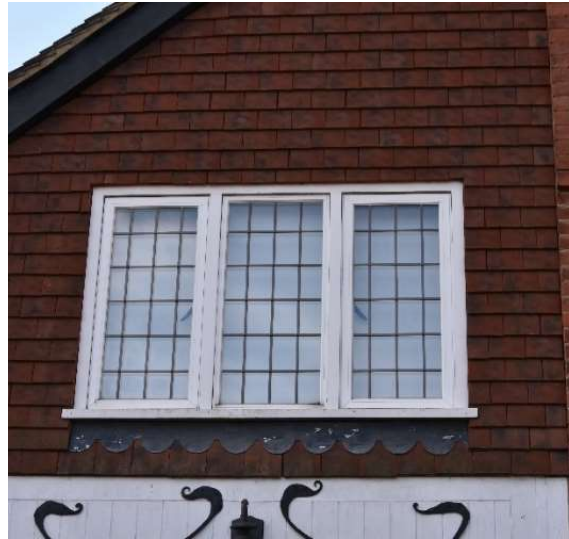
New timber and metal windows in 2009 Extension at No 9
