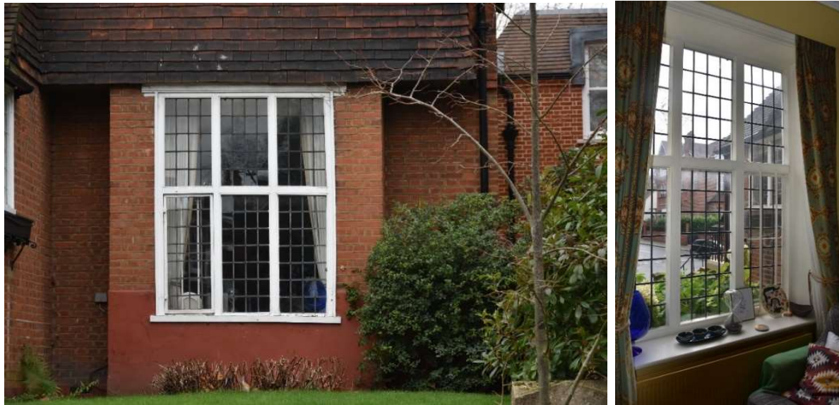
Single Glazed window to Dining Room external and Interior views.
