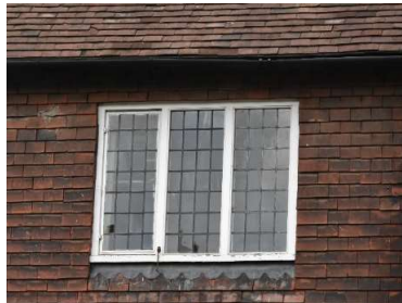
Single glazing 1 st Floor bedrooms exterior and interior views.
