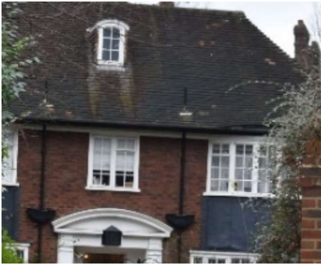
Existing timber windows in properties in Netherall Gardens
