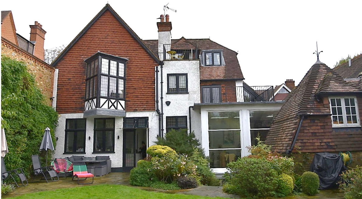
Rear elevation at No9 with typical Arts and Craft details with non-original double-glazed leaded windows in timber frame.
