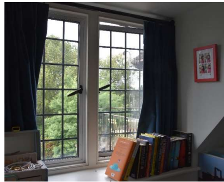
Double glazing to dormer window , single glazing to bedroom gable.
