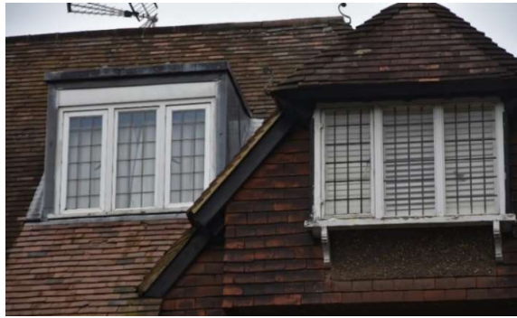
Double glazing to dormer window , single glazing to bedroom gable.
