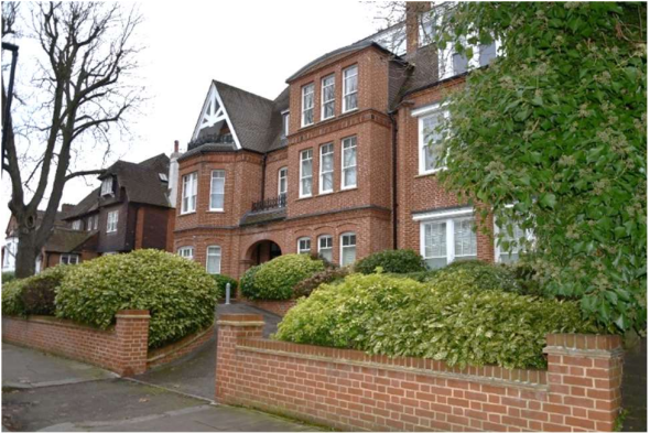
New build No11 Netherall gardens with No9 beyond.
