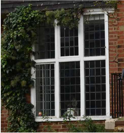
Single glazing: Top central panel replacement panel
