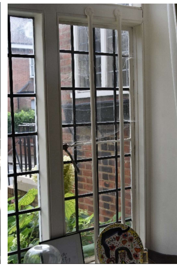
Ground fl. opening light security bars
