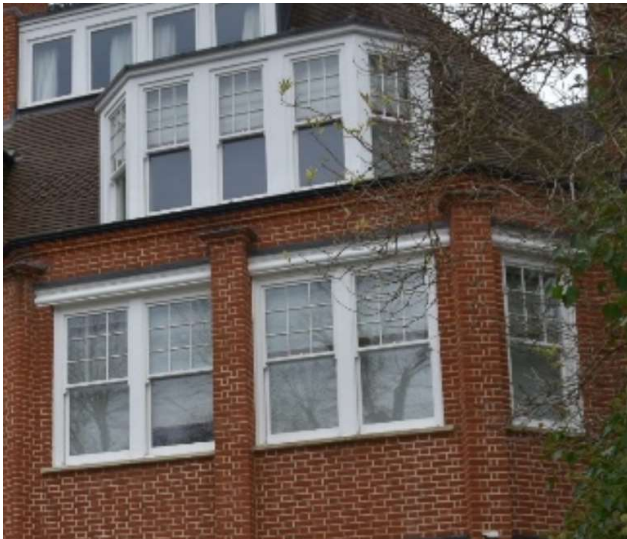
Timber windows in new building at No11
