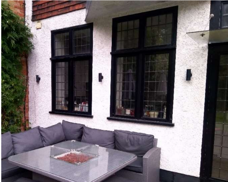
Double glazed Kitchen windows view
