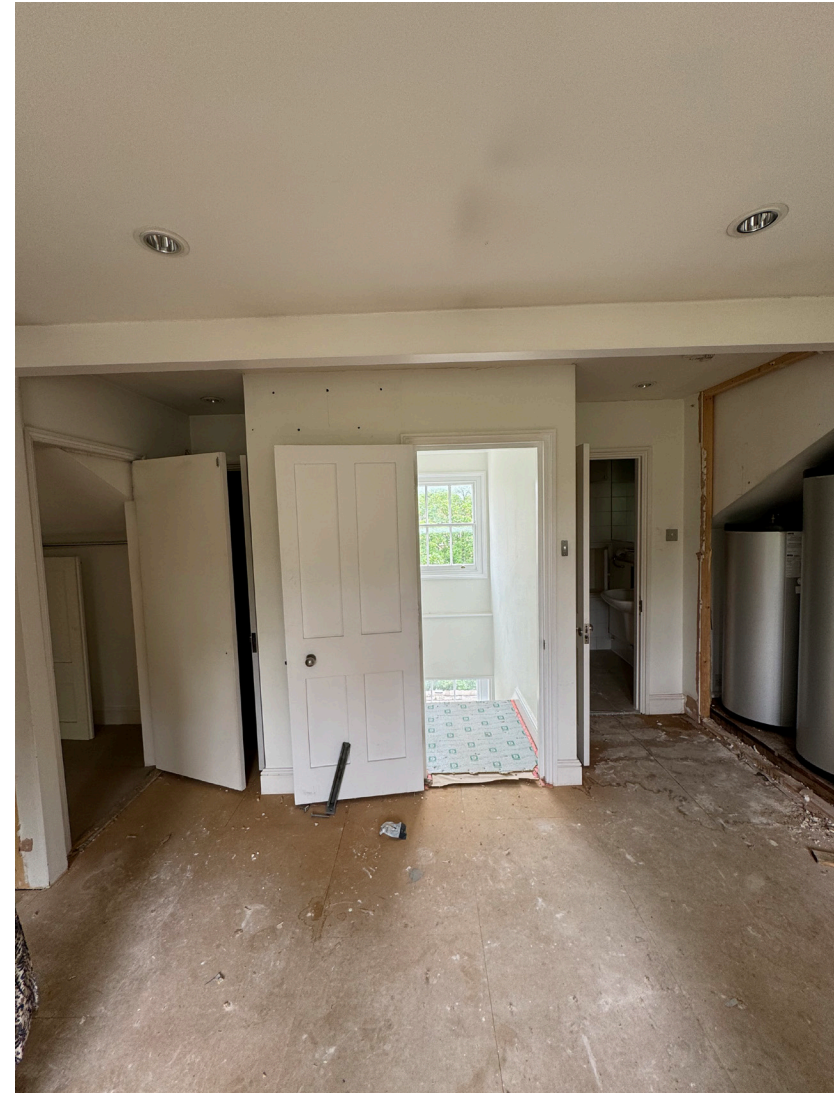
Existing third floor bedroom
