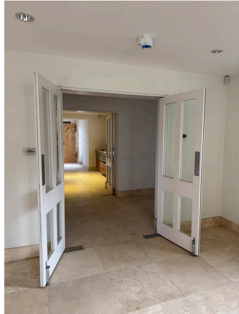
Existing ground floor family room door
