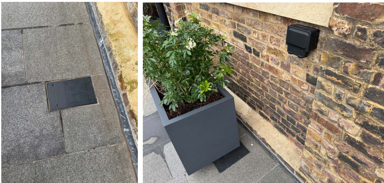
Fig 20: Existing floor and wall power and data outlets in the proposed site location are to be utilised to avoid any new services interventions
