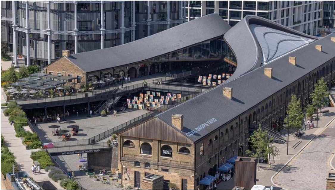
Fig 9: Aerial view of Coal Drops Yard today looking north-west, showing the enlarged southern yard and the sweeping new 'ribbons' at roof level. New bridges now link the historic viaducts.
