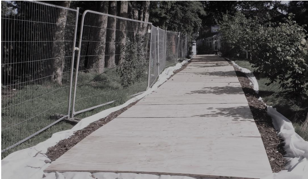
Figure 6: Ground Protection Example
