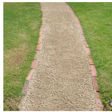
Somerset self binding gravel or equivalent
