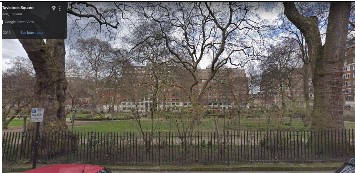
Google Street view: Tavis House, 1-6 Tavistock Square, front elevation view from across Tavistock Square gardens.
