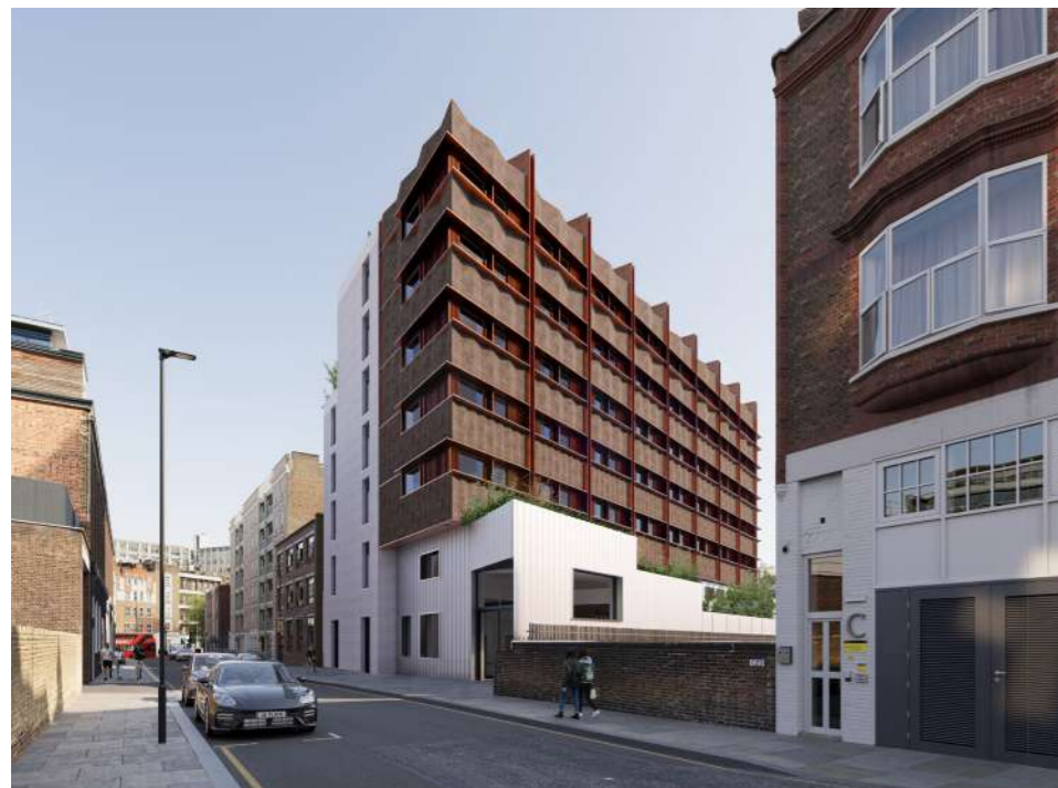
Figure 173 - A folded parapet - Tertiary feature becomes extremely prominent
