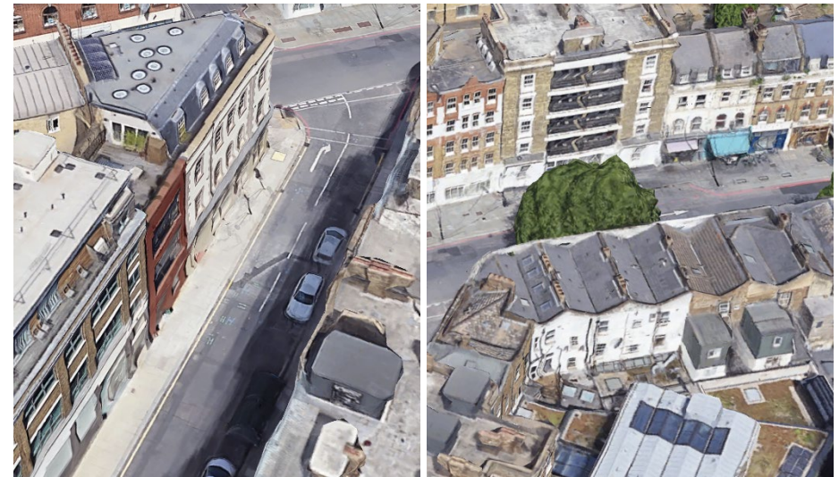
Figure E.2 – Satellite View (Google Earth) Images Showing Hard Surfaces and Cladding Within 10m of the Proposed Building to Help Score Question 9
