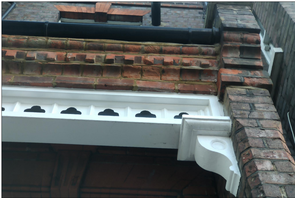
No. 22 Willoughby Road brick detail
