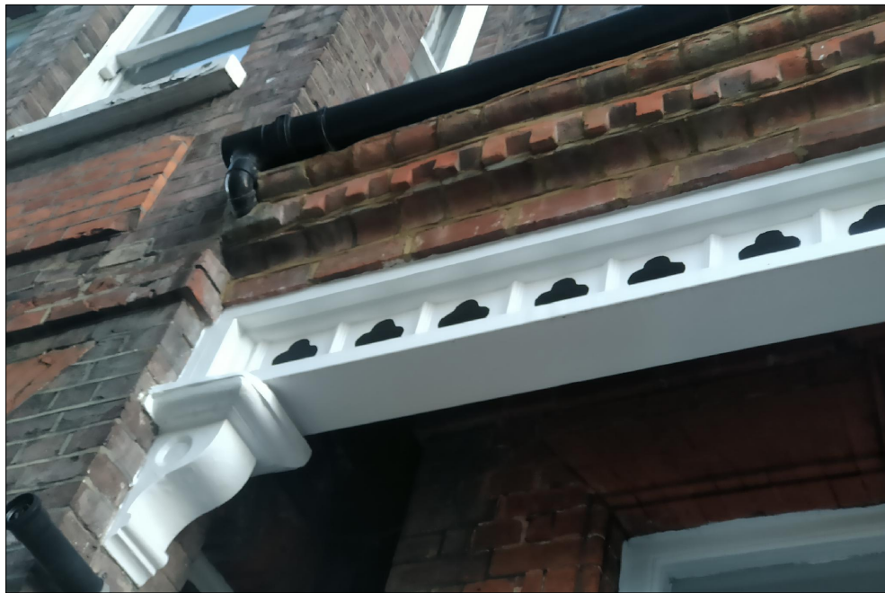
No. 22 Willoughby Road brick detail
