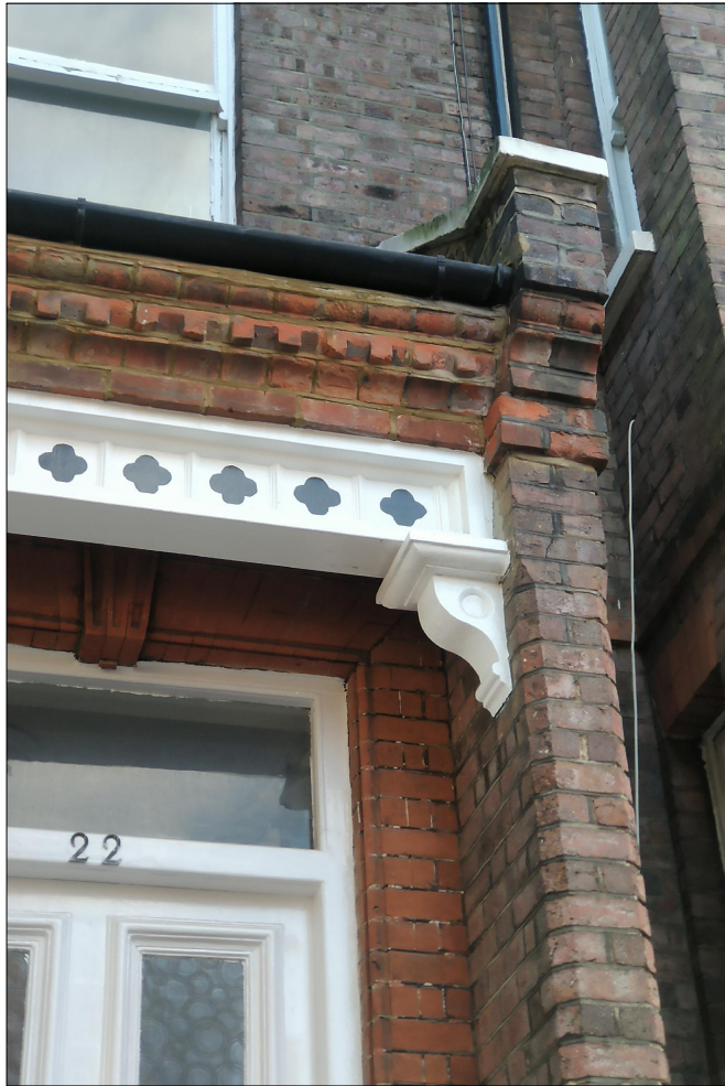
No. 22 Willoughby Road brick detail and coping stone at parapet wall
