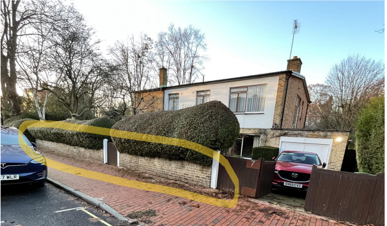
Above: Photograph showing the existing brickwork to the front boundary wall. It is proposed to rebuild the wall to the same size and dimensions, using the bricks approved for the main house under Application ref: 2024/5223/P. The proposed boundary brick wall would consist of the combined use of 'Chartham Multi Stock' randomly mixed through with 'East Barley Red Blend - dark red, and orange'
