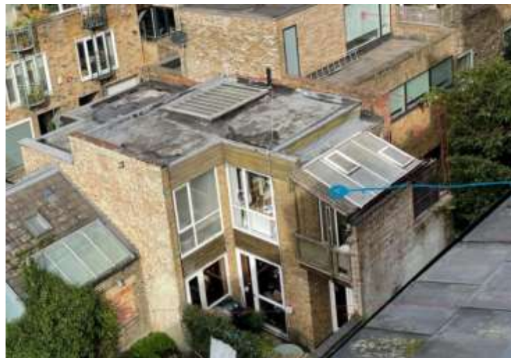
Aerial image of the rear of the site
