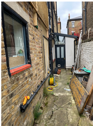
Boundary wall with fencing
