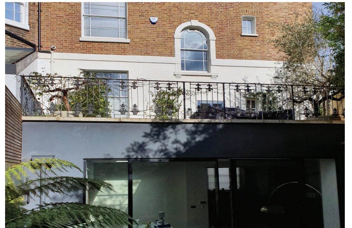
← Opposite boundary wall, as seen from lower ground level
