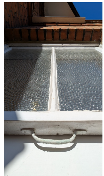
exterior view of outer sash
