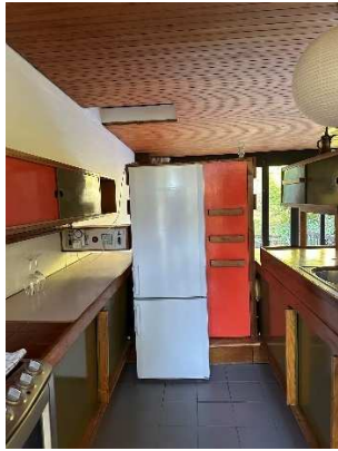
Figure 6 - Full height fridge which does not fit comfortably in cupboard
