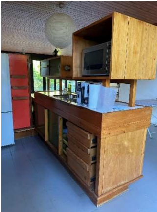
Figure 8 - Excessively large high-level unit for microwave
