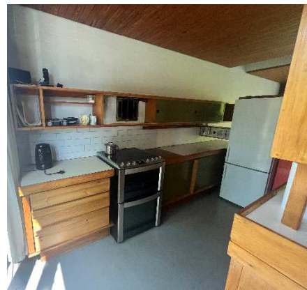
Figure 9 - Existing oven protrudes past worktop. Formica door fronts use sliding mechanisms.
