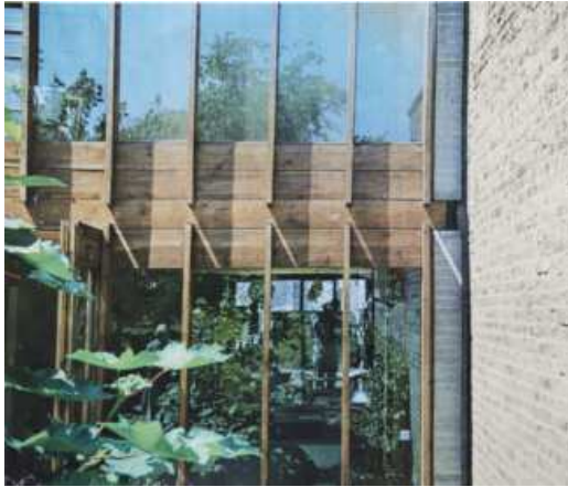
Figure 1- Original cladding tone - Modern House date unknown
