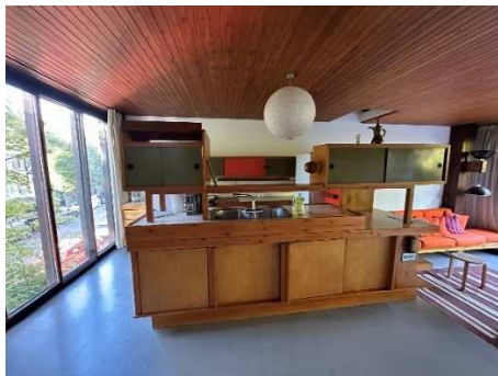
Figure 5 - Kitchen long elevation with swing doors at low level and raised sink worktop
