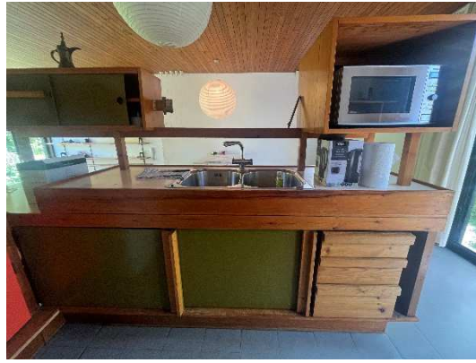
Figure 7 - Sink worktop. High level units have sliding doors or are open shelves. Low level sliding doors to cabinets and pull-out drawers RHS
