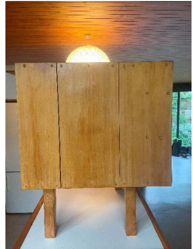
Figure 13 - Timber dowels do not follow a setting out pattern
