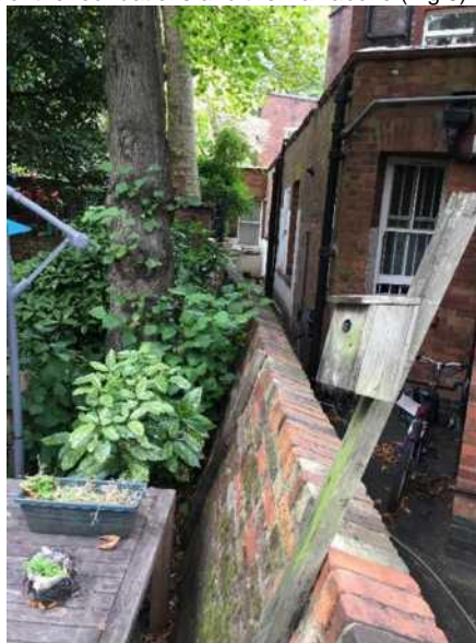
Fig 7. Wall between No.10 and 58. Facing No. 12 with No. 58 to the right. Mature tree within the garden of No. 10 and wall leaning significantly towards No.58
