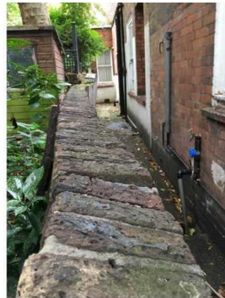
Fig 7. Wall between No.10 and 58. Facing No. 12 with No. 58 to the right. Mature tree within the garden of No. 10 and wall leaning significantly towards No.58
