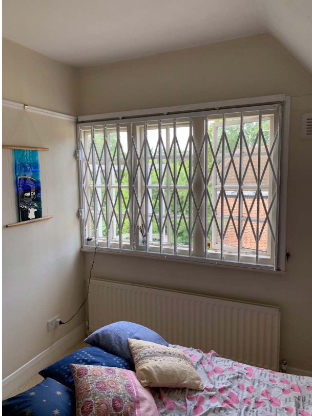
Figure 16 Photograph of the existing rear elevation 4-partite window as seen from inside.
