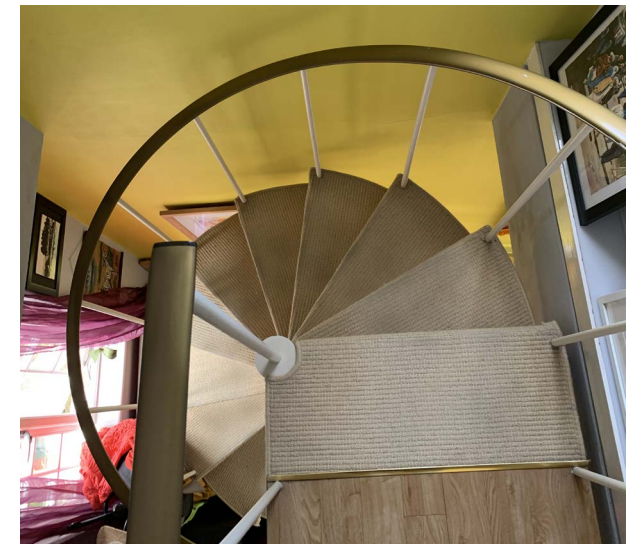
Figure 22 Photograph of the existing spiral staircase to be replaced.
