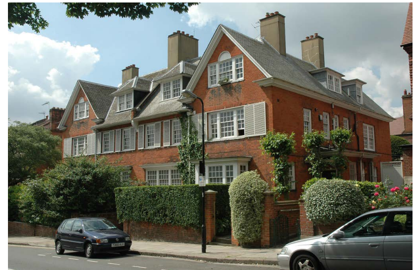
Figure 20 Modern photograph of No.51 Frognal.
