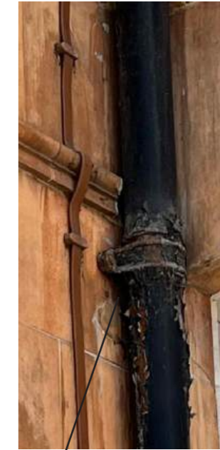
Replacement of damaged rainwater goods
