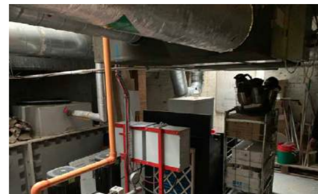
Lower ground plant space west with pavement lights
