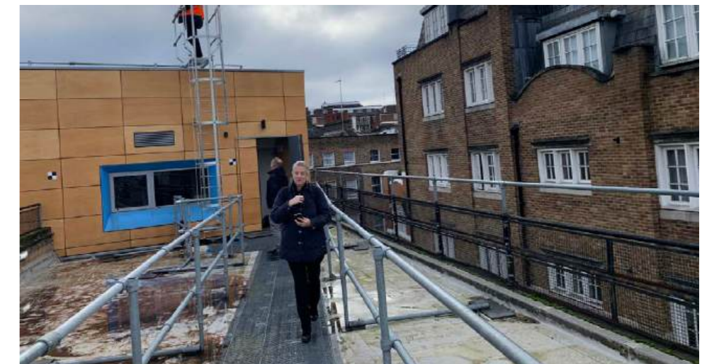
15. Lower roof looking south
