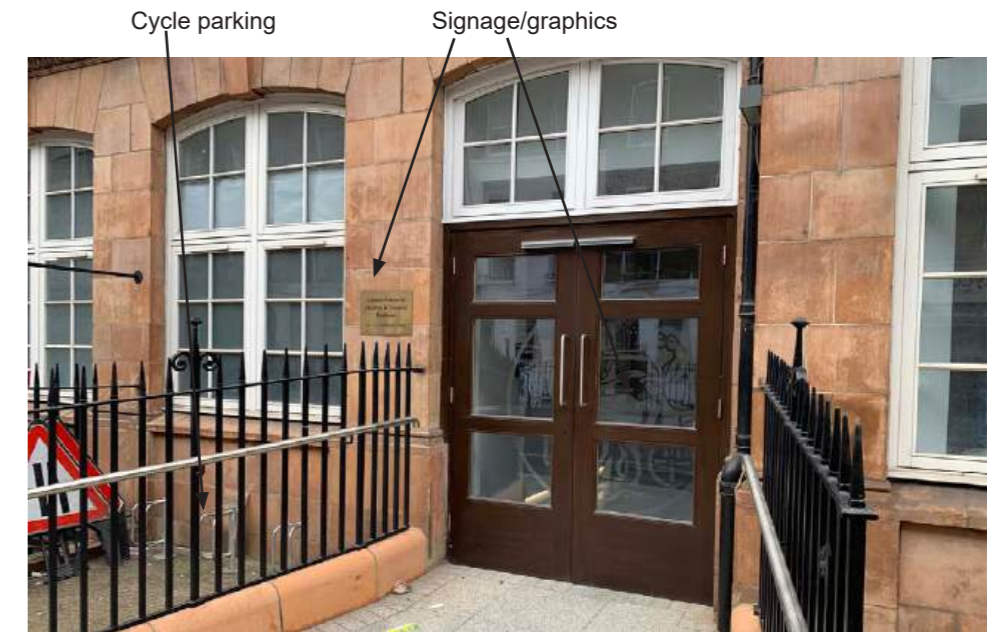
8. TP1 eastern end current (temporary) main entrance
