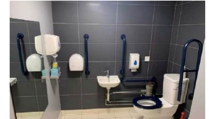
Lower ground wc
