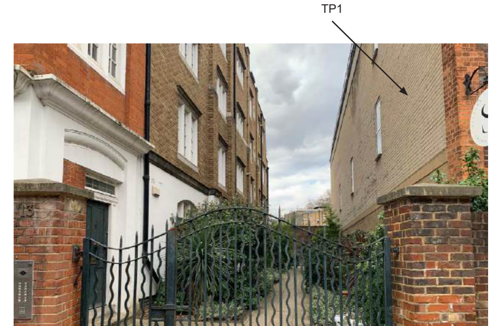
2. Western end of TP1 and adjacent property
