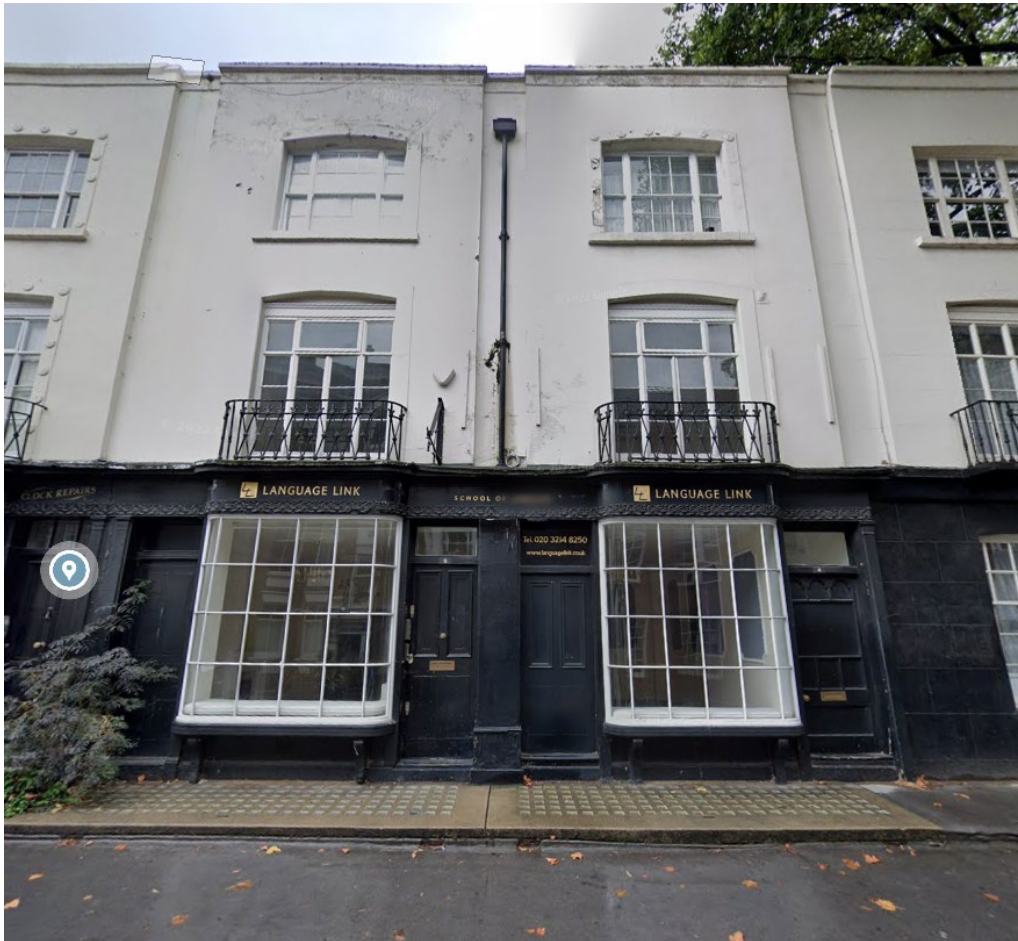
Google Street view of the property frontage.
