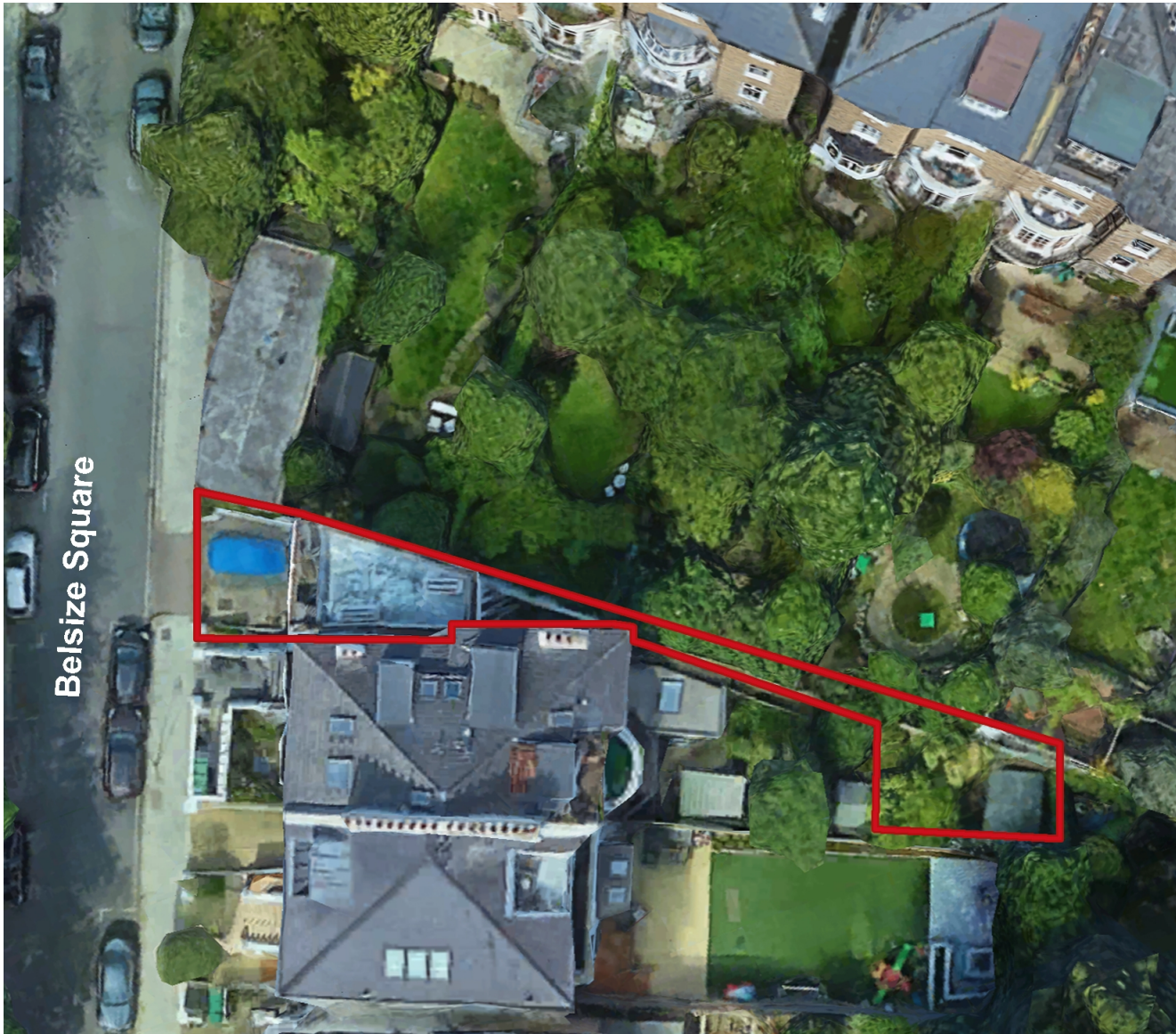
Fig. 1 Aerial view of The Coach House, 50A Belsize Square, NW3 4HN.
