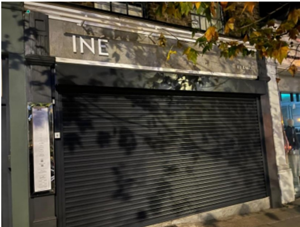
Figure 1 – Photograph of Hampstead High Street shutter
