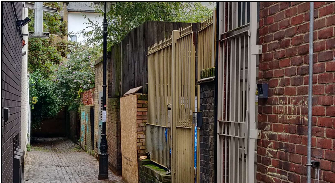
Existing boundary treatment
