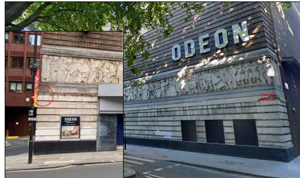
FIG.2 / FIG.3 - STREET-VIEW PHOTOGRAPH OF SUBJECT ELEVATION / CLOSE-UP OF PROPOSED INVESTIGATION AREA A. NOTE: SWL RED ANNOTATION SHOWS PROPOSED LOCATIONS FOR INITIAL INVESTIGATIONS.
