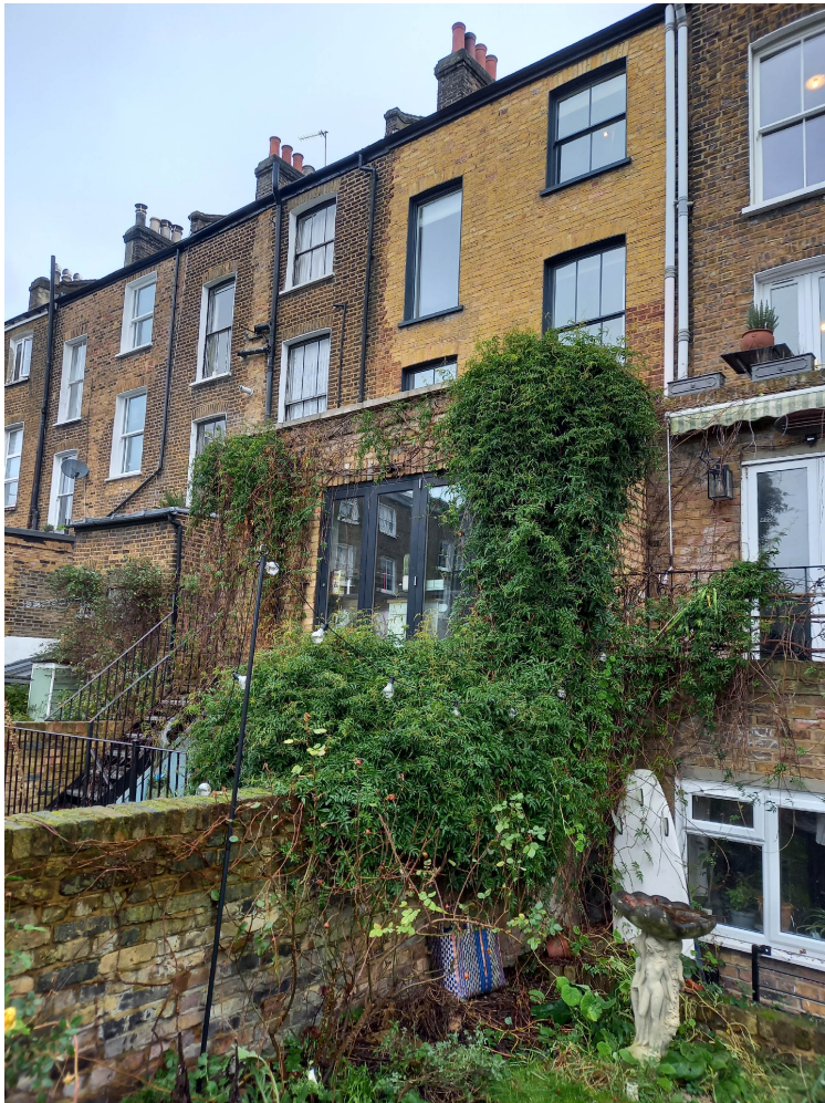
View of rear extension to no 27
