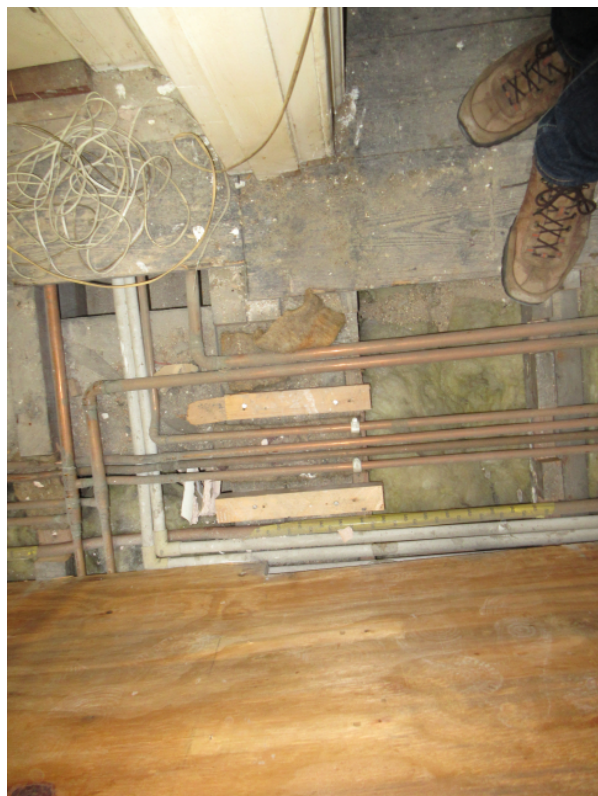
Floor beam at spine wall.
