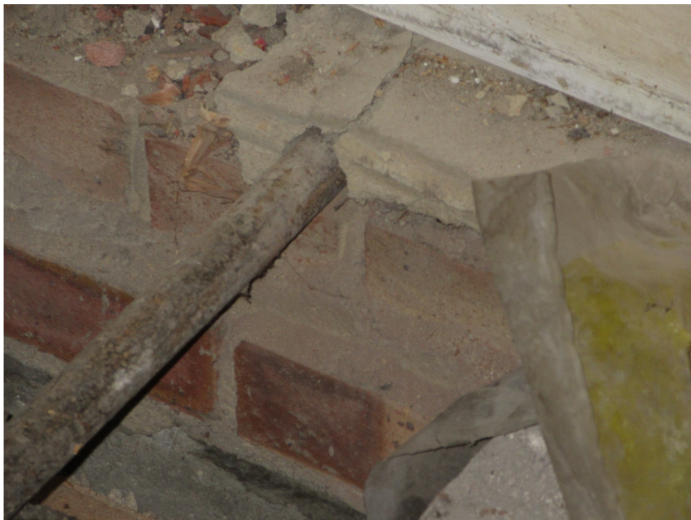
Tie bar at front wall.
