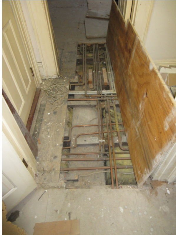
Floor beam to bedroom at spine wall.
