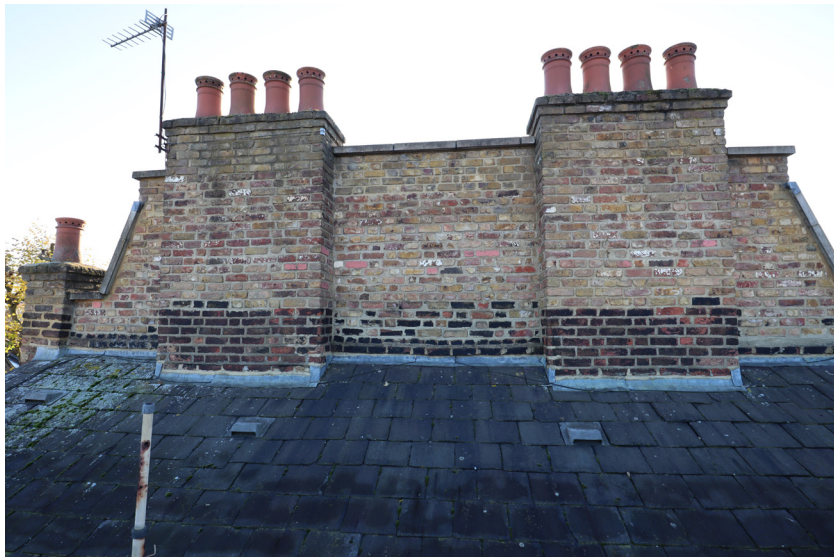
Existing party wall with 40 Gayton Rd and butterfly roof Gayton Road
