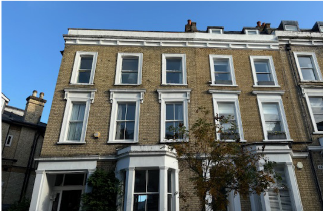
Existing Front Elevation - mansard roof extensions at 40 and 41 Gayton Rd visible
