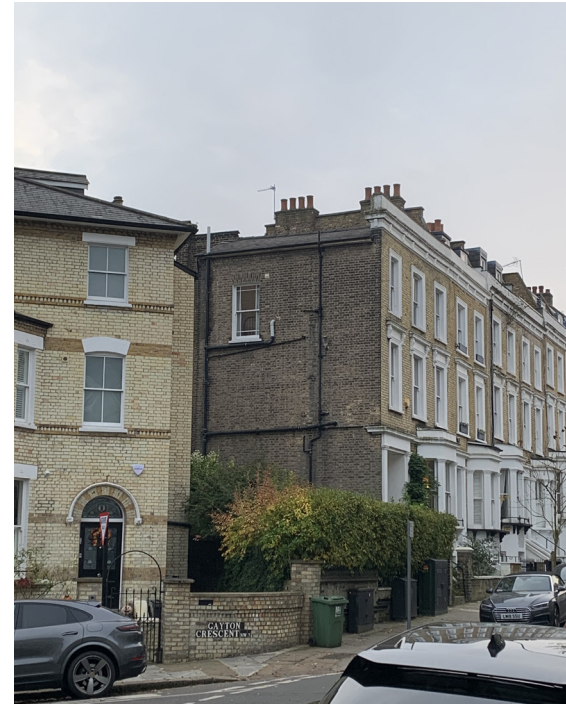
Existing Side Elevation and 1 Gayton Crescent (LHS of photo)
