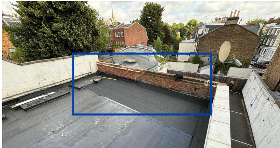
Flat roof – looking away from building The blue outline indicates the proposed plant location
