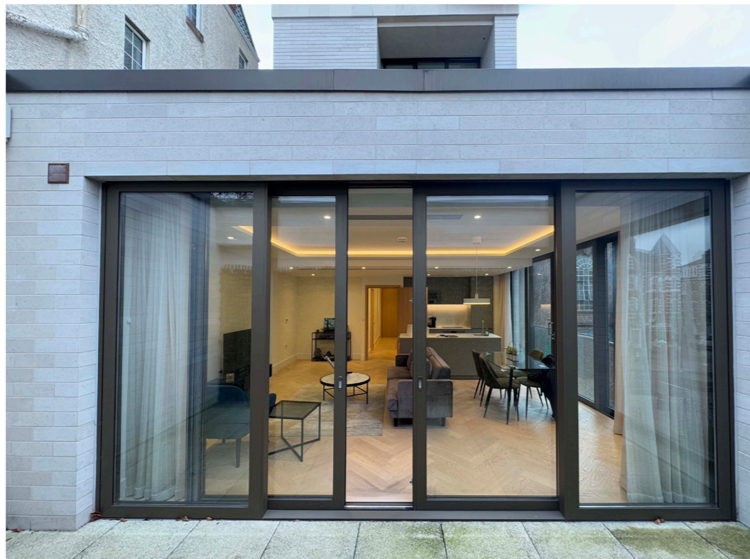
192 Haverstock Hill - Existing Sliding Screen To Flat 2 Lightwell
