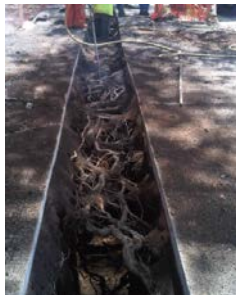
Example imagery of air spade use for implementing utilities beneath root plate (existing)
