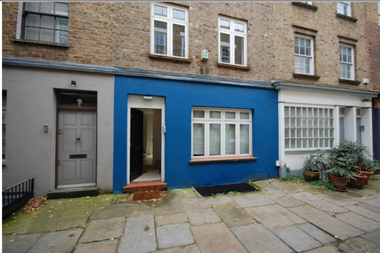
FRONT NORTH WEST FACING ELEVATION
