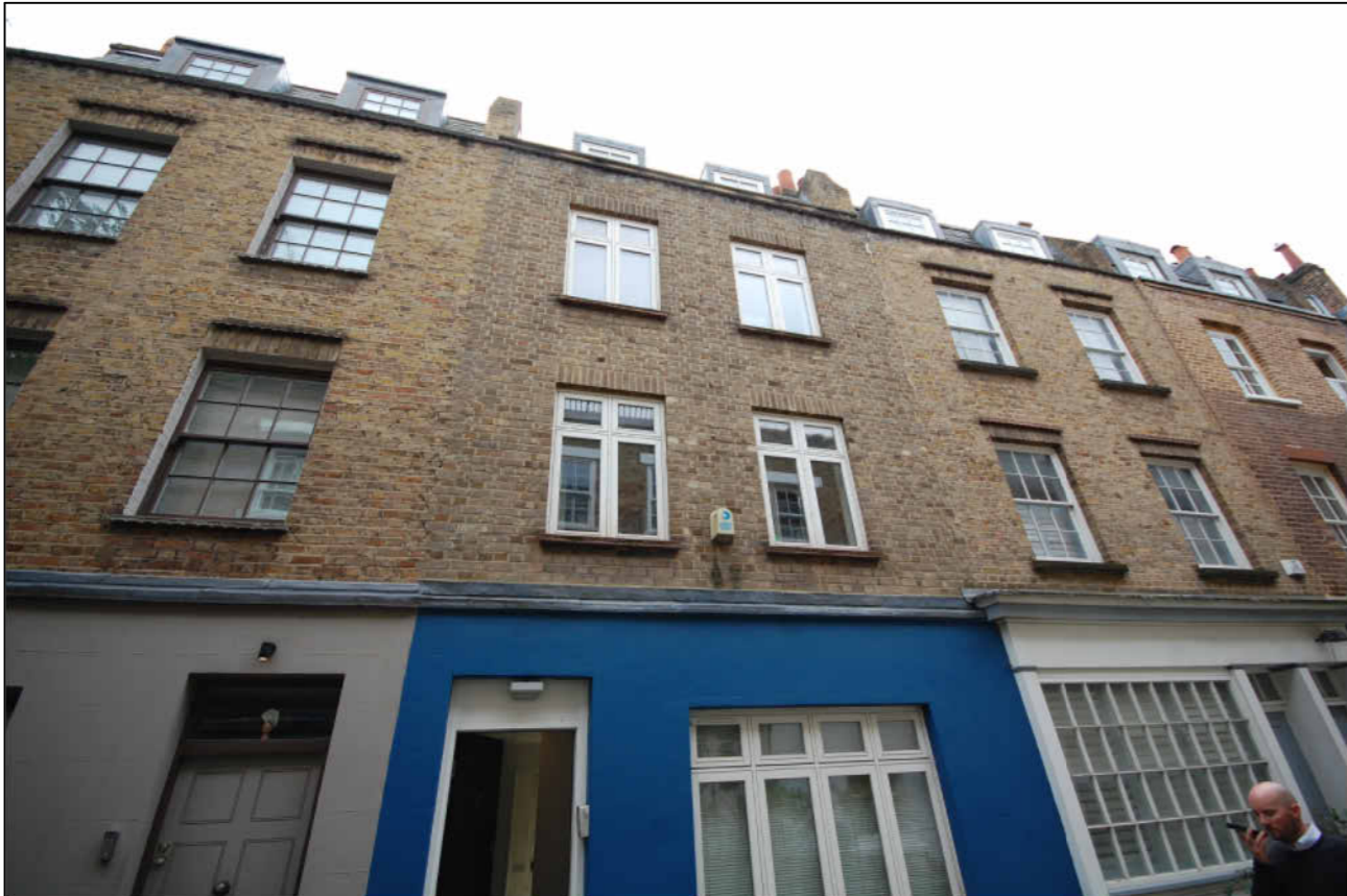
FRONT NORTH WEST FACING ELEVATION
