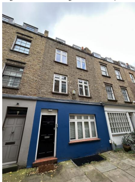
Figure 2 and 3: Existing front and rear photos
