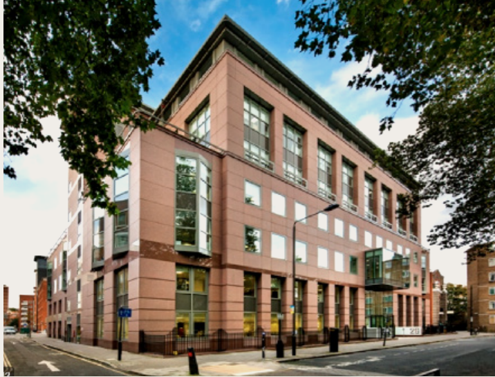
Existing Red Lion Square / Old North Street view
