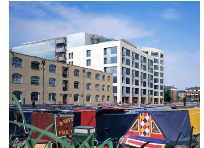
Example of AVR 3 – confirming the use of materials (in this case using a ‘photo-realistic’ rendering technique)
