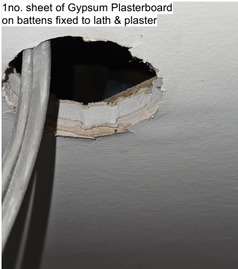
1no. sheet of Gypsum Plasterboard directly fixed to lath & plaster
