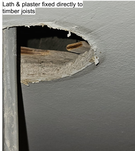
1no. sheet of Gypsum Plasterboard directly fixed to lath & plaster
