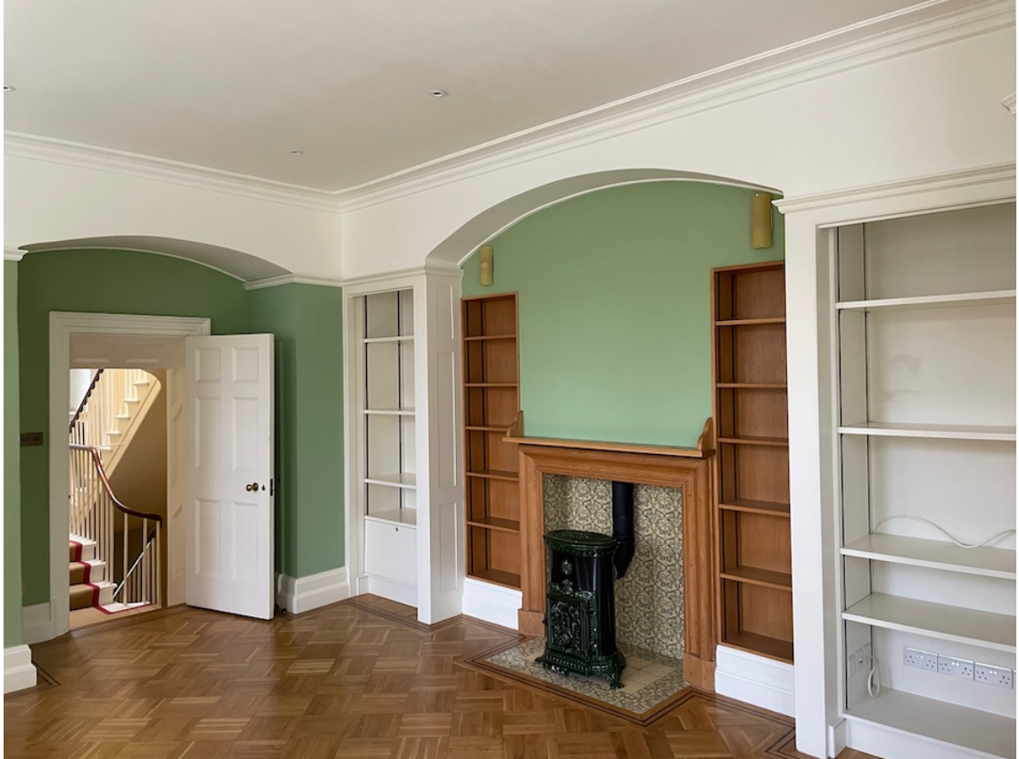
Remove non-original shelving, suspended ceiling & spotlights
