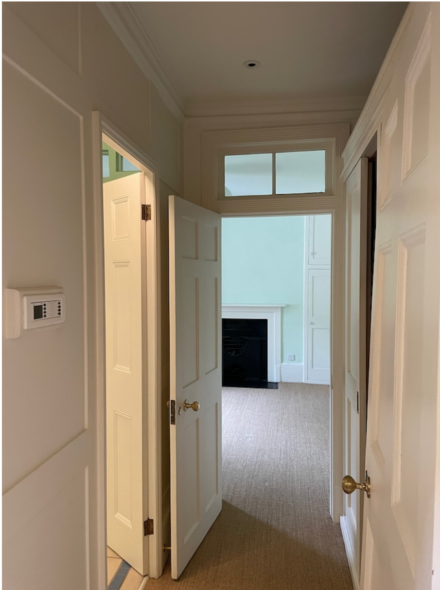
Non-original internal rooms to be removed along with suspended ceilings & spotlights
