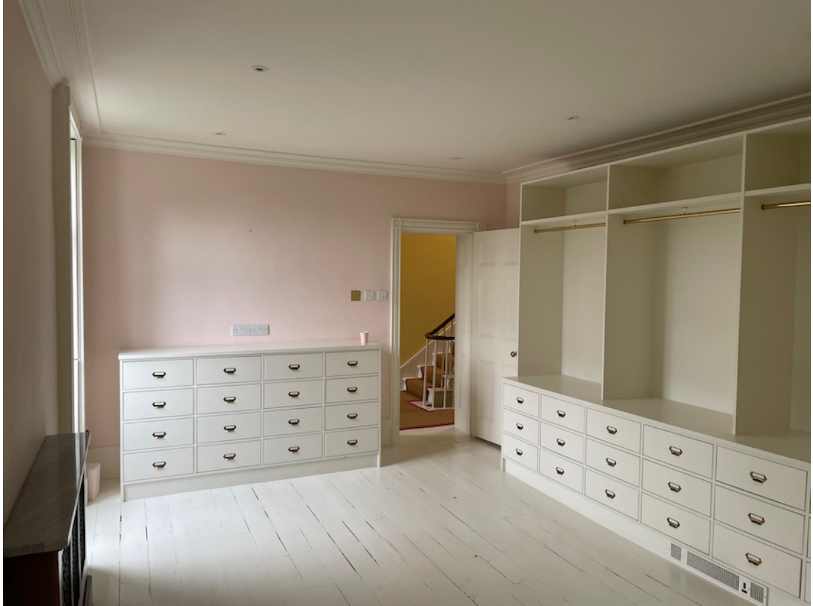
Remove non-original suspended ceiling & spotlights: create new double door opening
