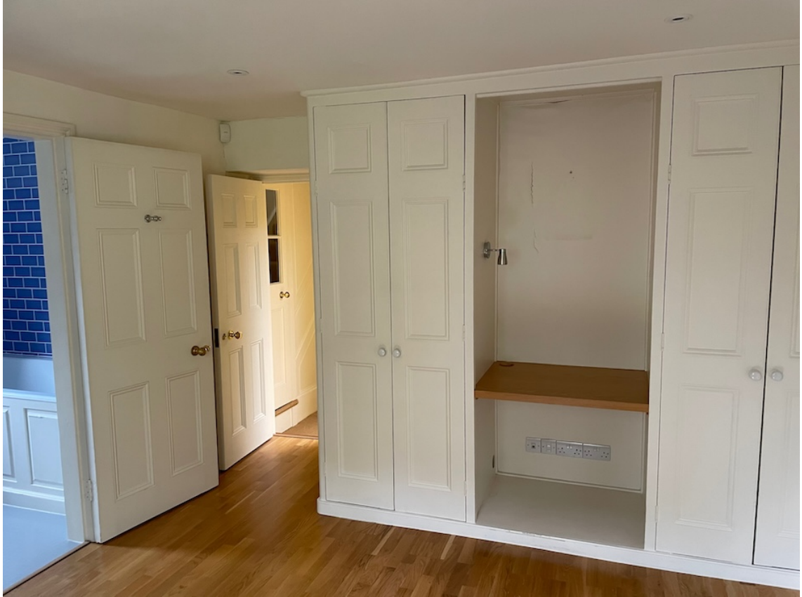
Original 'tower' room to reinstated; suspended ceiling spotlights removed
