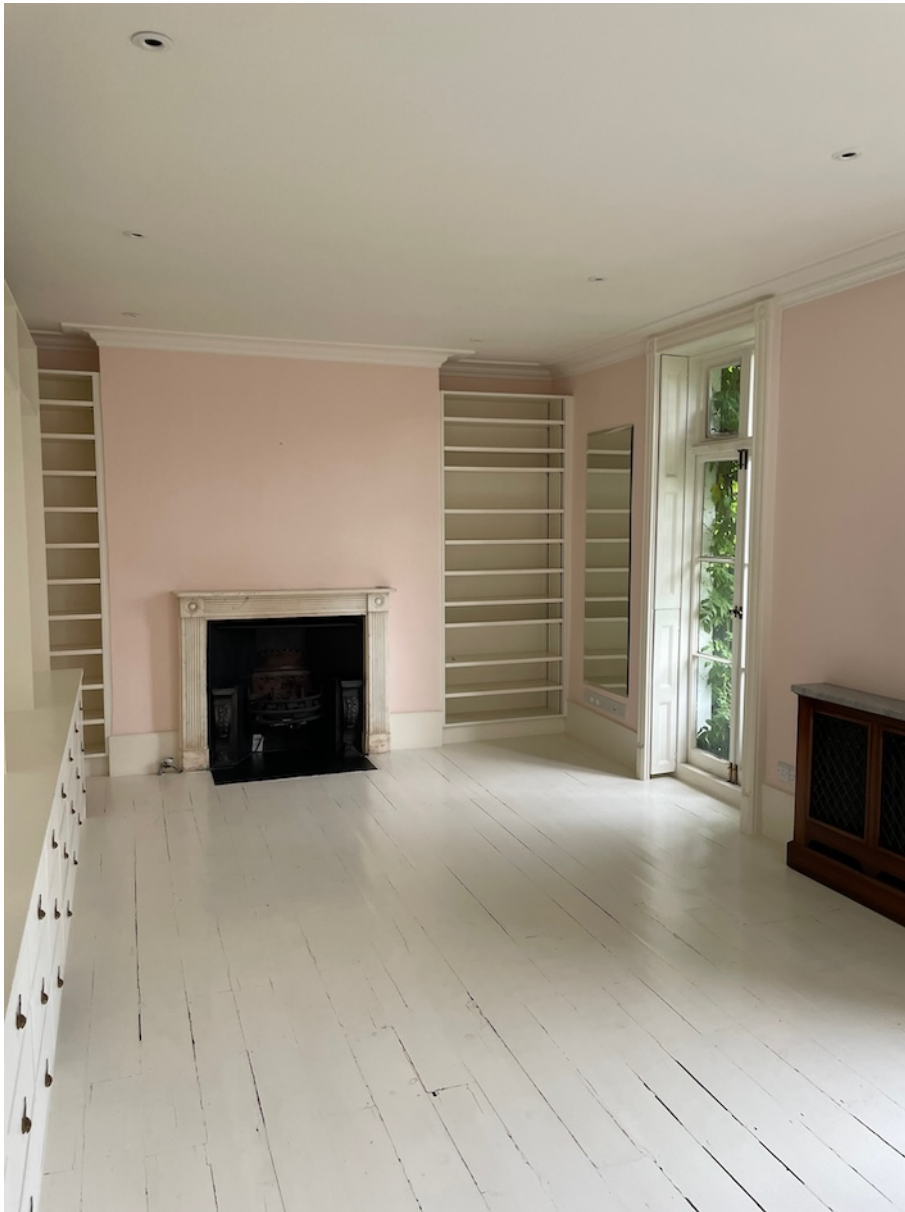
Remove non-original suspended ceiling & spotlights: create new double door opening
