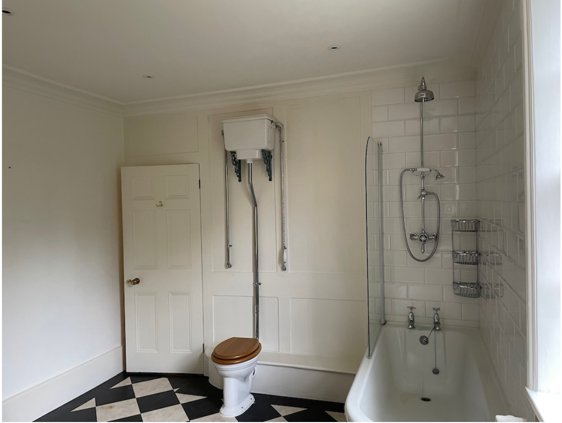
Sanitaryware and plumbing to be removed
