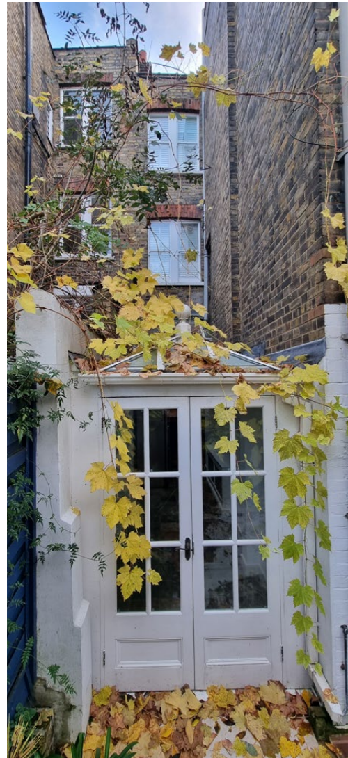
View of existing rear infill extension
