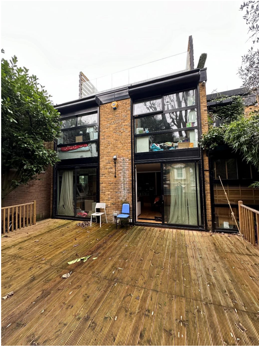
Figure 4 Rear elevation (Source: site visit)
