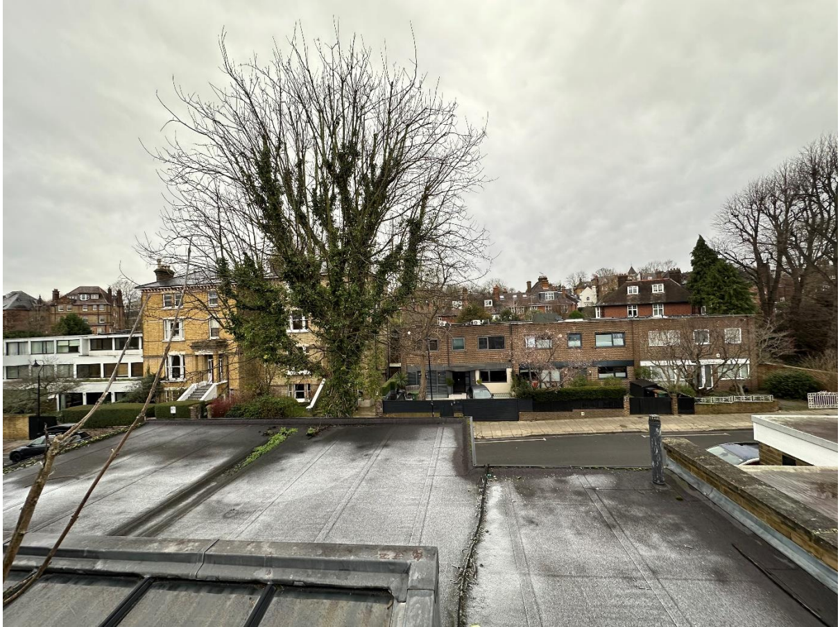
Figure 11 Existing flat roof towards the front (Source: site visit)
