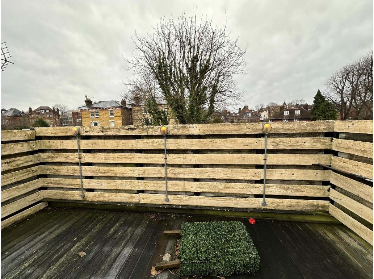
Figure 10 Existing roof terrace (Source: site visit)
