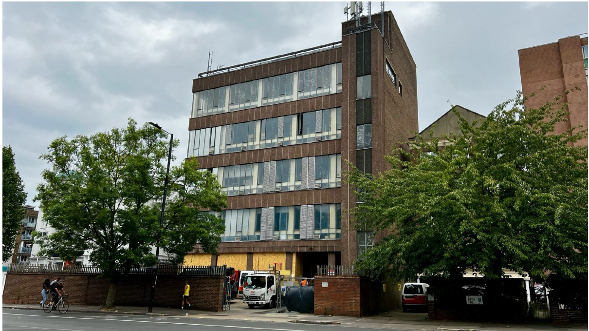
Figure 7 – View of Maida Vale TE Frontage
