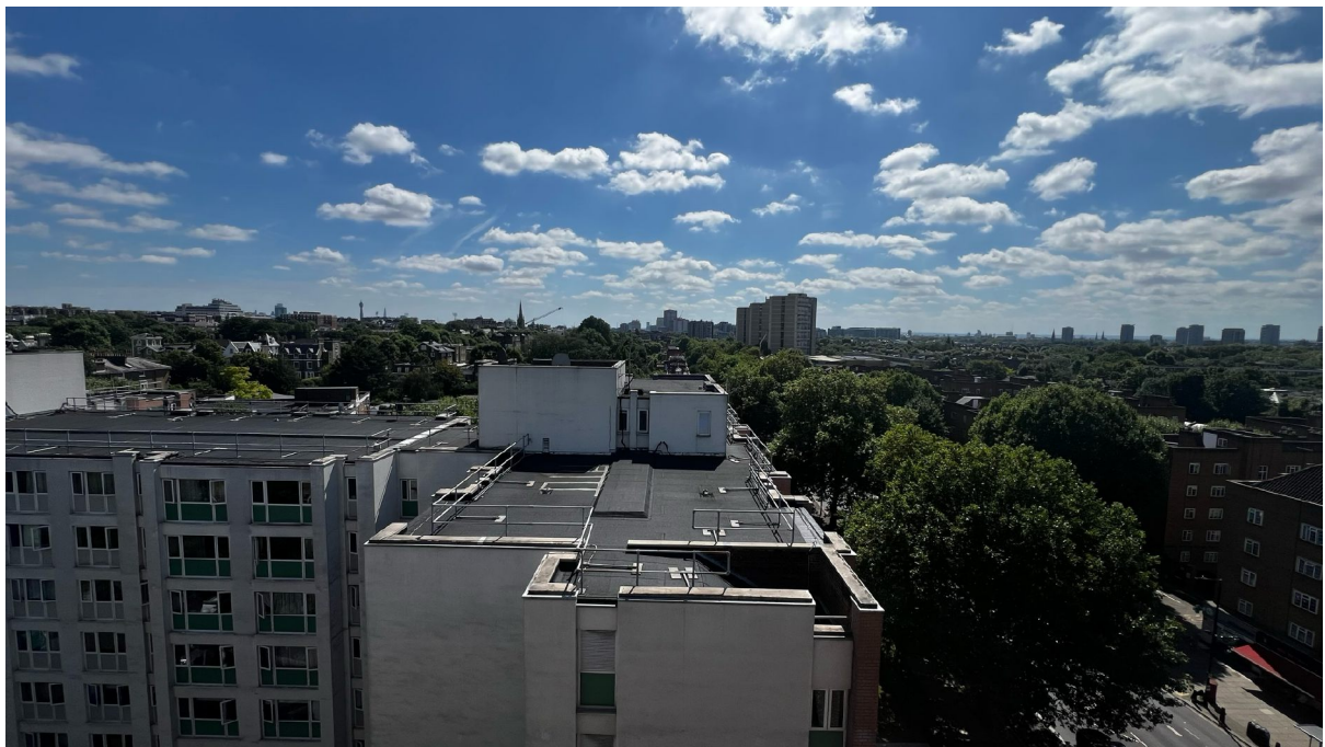
Figure 8 – View towards South-East Receivers Adjacent (Taken from 6 th Floor Roof)
