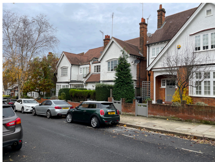
Street view, no. 25 centre.
