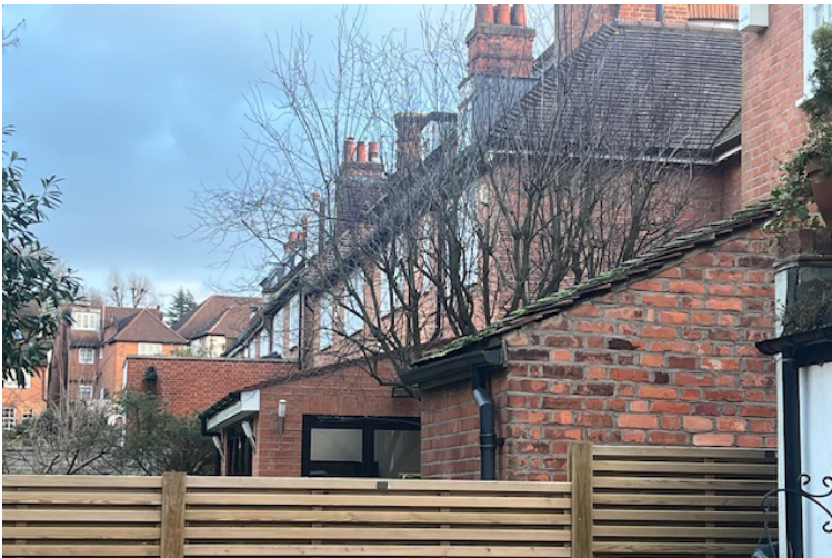
The rear extensions of nos. 21 & 23.
