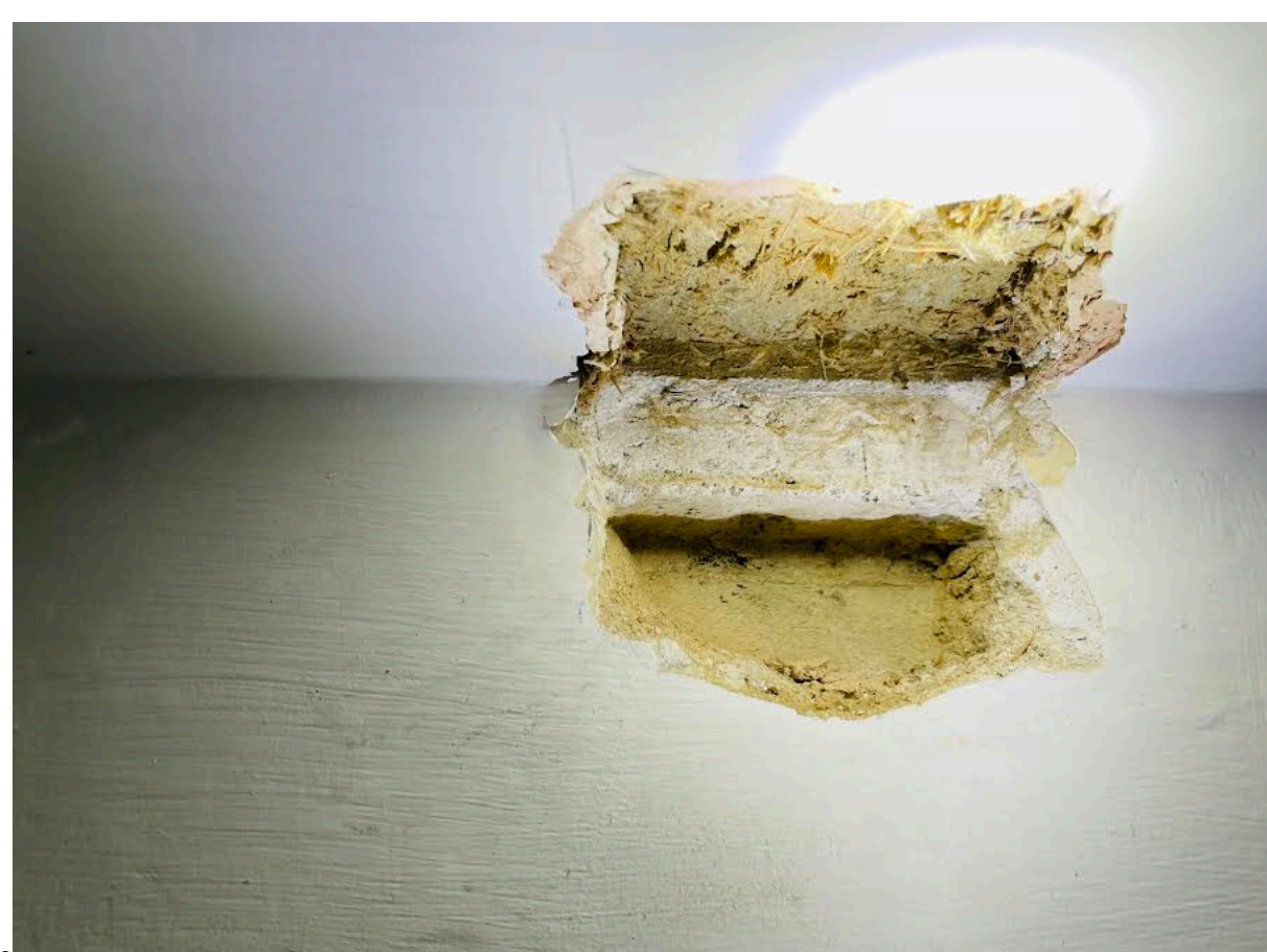
Photo of wall between toilet and bathroom
