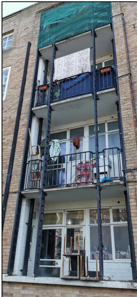
Photo 2: External view of inset balcony
