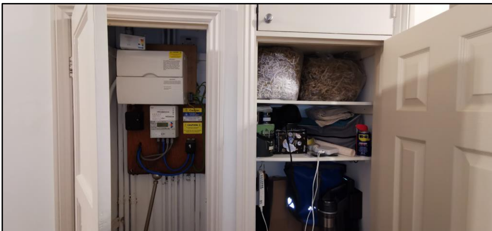
Photo 4: Openings to cupboards in corridor wall on kitchen side
