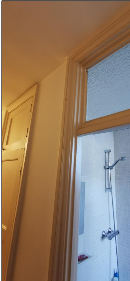
Photo 7: Wall between corridor and bathroom proposed to be removed
