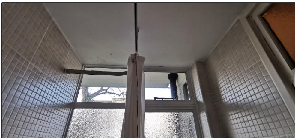
Photo 9: Front wall of bathroom overlooking inset balcony
