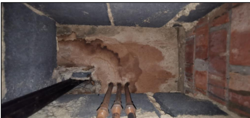
Photo 5: Wall structure visible above electrical cupboard
